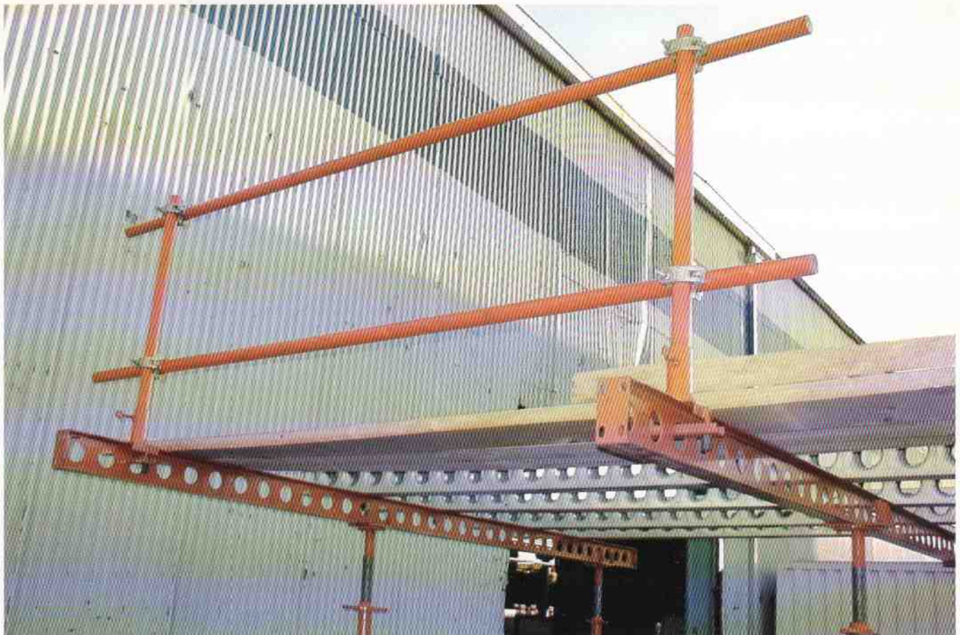
TYPICAL CANTILEVER PROTECTION DETAIL
